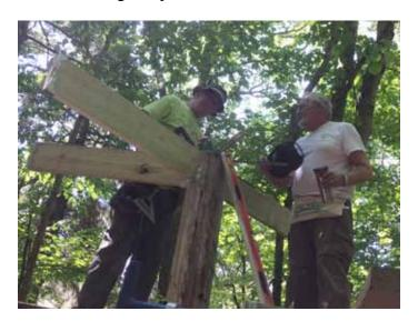
Jerry had roughly pre-cut most of the lumber and numbered all the pieces in order of assembly, so we were able to make quick progress on this build. Here we have added diagonal 2X6 supports to stabilize the stringers all around the pole.
