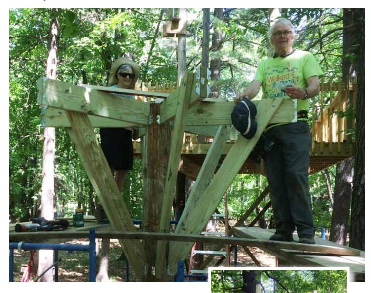
Kathy was right up there with Rick installing bolts and screws, so it wasn't long before we had 4x4 posts attached to the corners of the hexagon!
